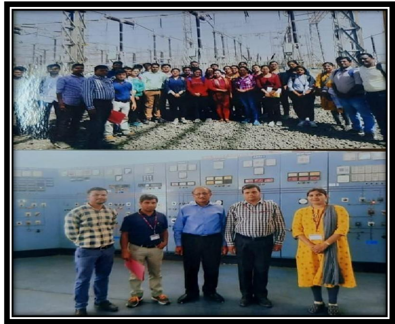
MPEB 400 Kv Substation
